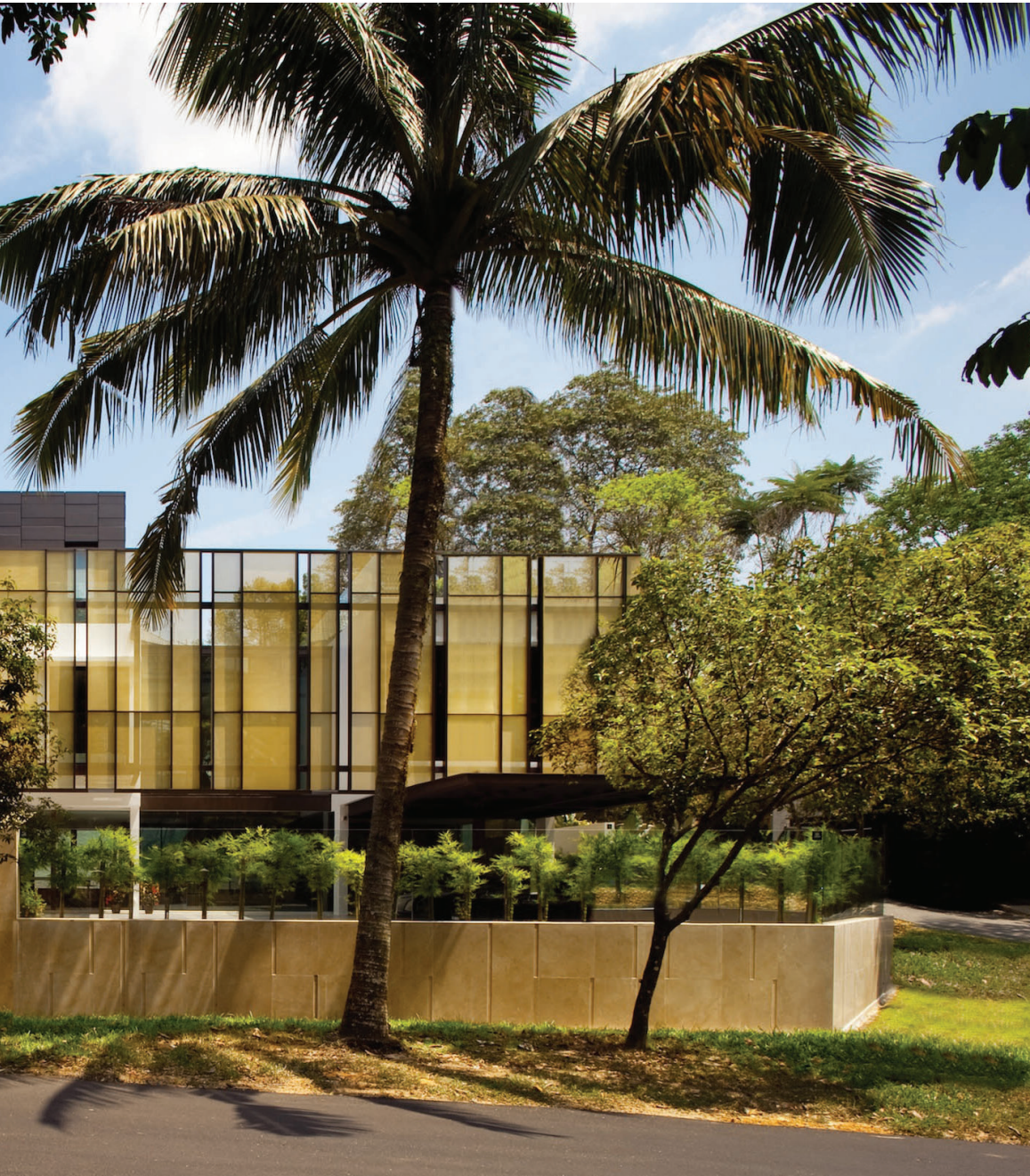
In the Golden Box house, metal was used as a mesh, veiling the building façade to dematerialise the volume and scale.
