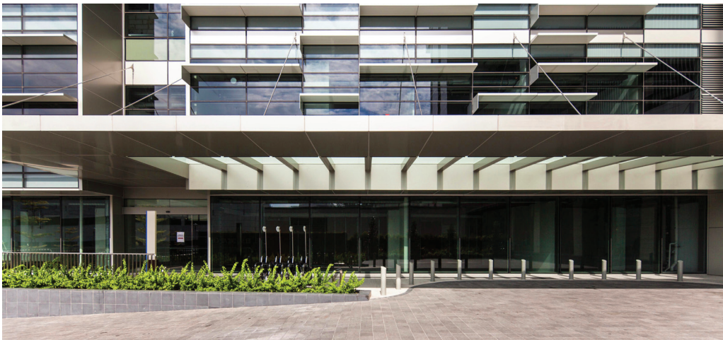
The National University Hospital entrance has deep canopies that are a contemporary interpretation of classic equatorial architectural elements. The façade design has been proven to provide up to 75 percent of shade annually.
