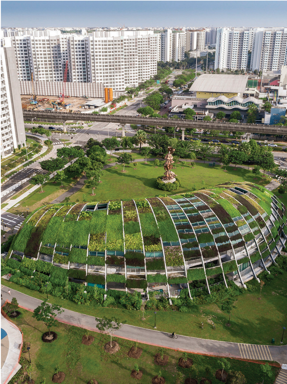
Sengkang Riverside Park Preschool has a green roof supported by steel ribs designed using advance computer software to arrive at this final structure.
