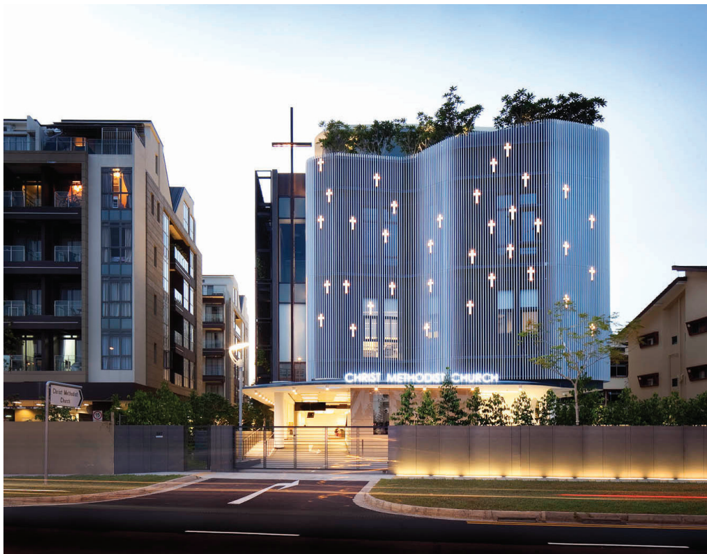
A simple, singular, rectangular aluminium extrusion was used to create the veiled façade of Christ Methodist Church.
