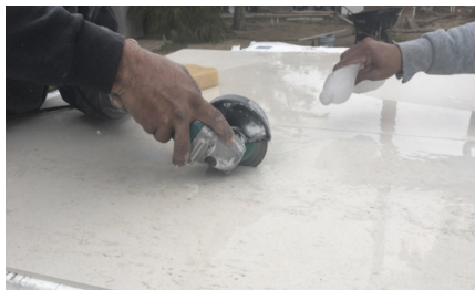
Straight cut with disc and water supply
