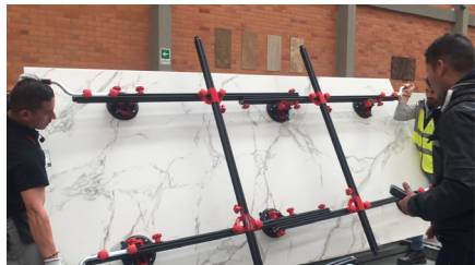
Handling with suction cups for large-format pieces
