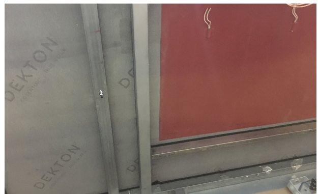
6.2.3. Support distance greater than 5 cm (2").
