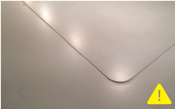
6.5.1. Potential chip on non-rounded edges on flush mounted plates.
