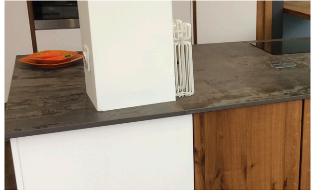
1.4.2. Integration of a pillar in a buffet through joints and L-piece.
