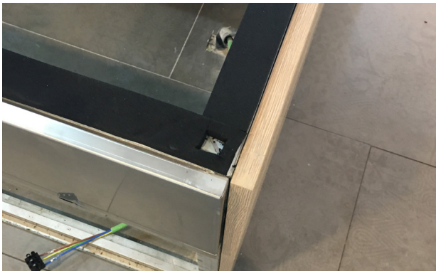
3.1.8. Leave gaps for fixing points.
