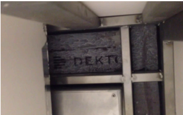
2.2.2. Cut-outs larger than 25x25 cm (10" x 10") will have continuous support under the 4 sides.
