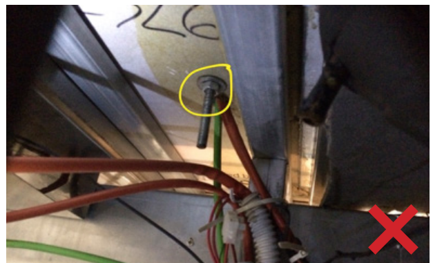
4.3.4. The screen post cannot be fixed to the countertop.
