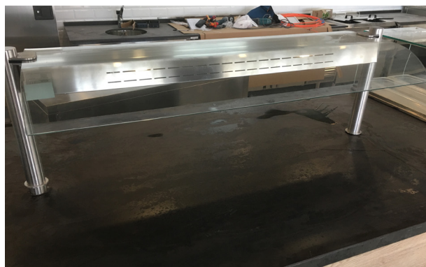
4.1.5. The screen post does not stress the countertop. Wear a trim that covers the drill.
