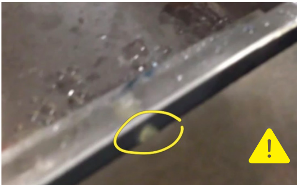
1.8.3. Hot appliances must have a separator between the Dekton and the appliance.
