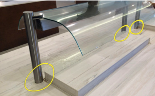
4.2.1. The screen post is badly located (in a corner) and does not respect the minimum distance.
