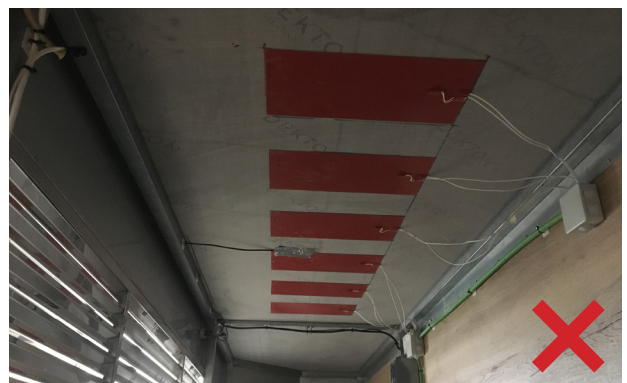
6.6.4. Missing casing and insulation. Poor temperature sensor placement.
