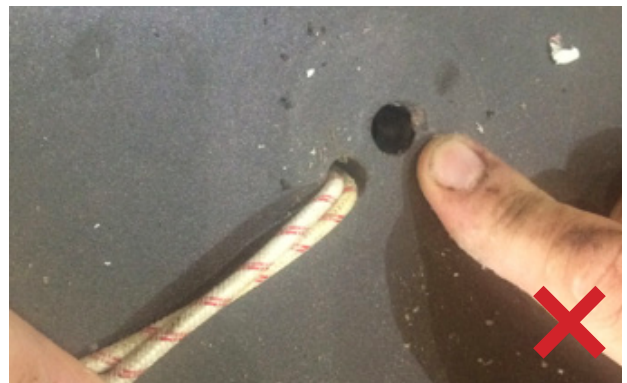
4.3.3. No more than one drill hole per screen post is allowed.
