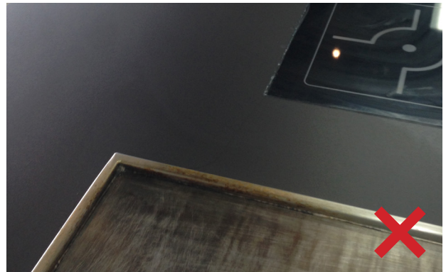
1.9.3. No recesses are allowed on the edge for food service and industrial kitchen applications (they are allowed for domestic countertop applications).
