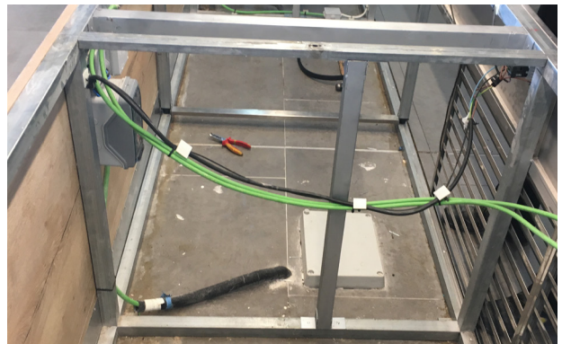
2.2.4. Example of upright frame to unload the efforts due to the attachment of a screen.
