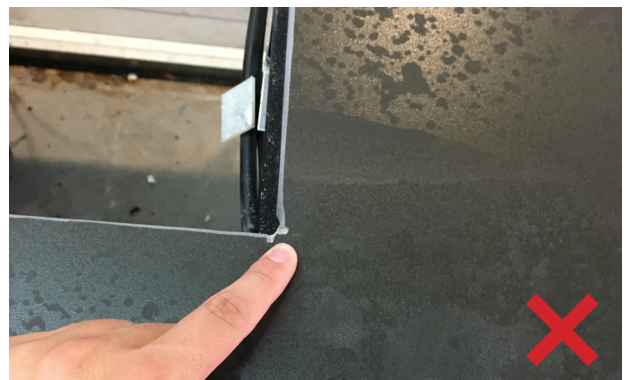
1.9.4. Radius made with discs.
