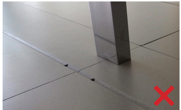
5.4.2. Drain holes are traditional in materials such as granite but in Dekton they are not advised. Dirt around involves health risks and food that does not compensate for water collection once the cold production equipment is turned off.
