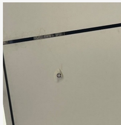
Pictures with examples of chippings produced by water penetration into the drills, combined with freezing temperatures, causing the product breakage.
