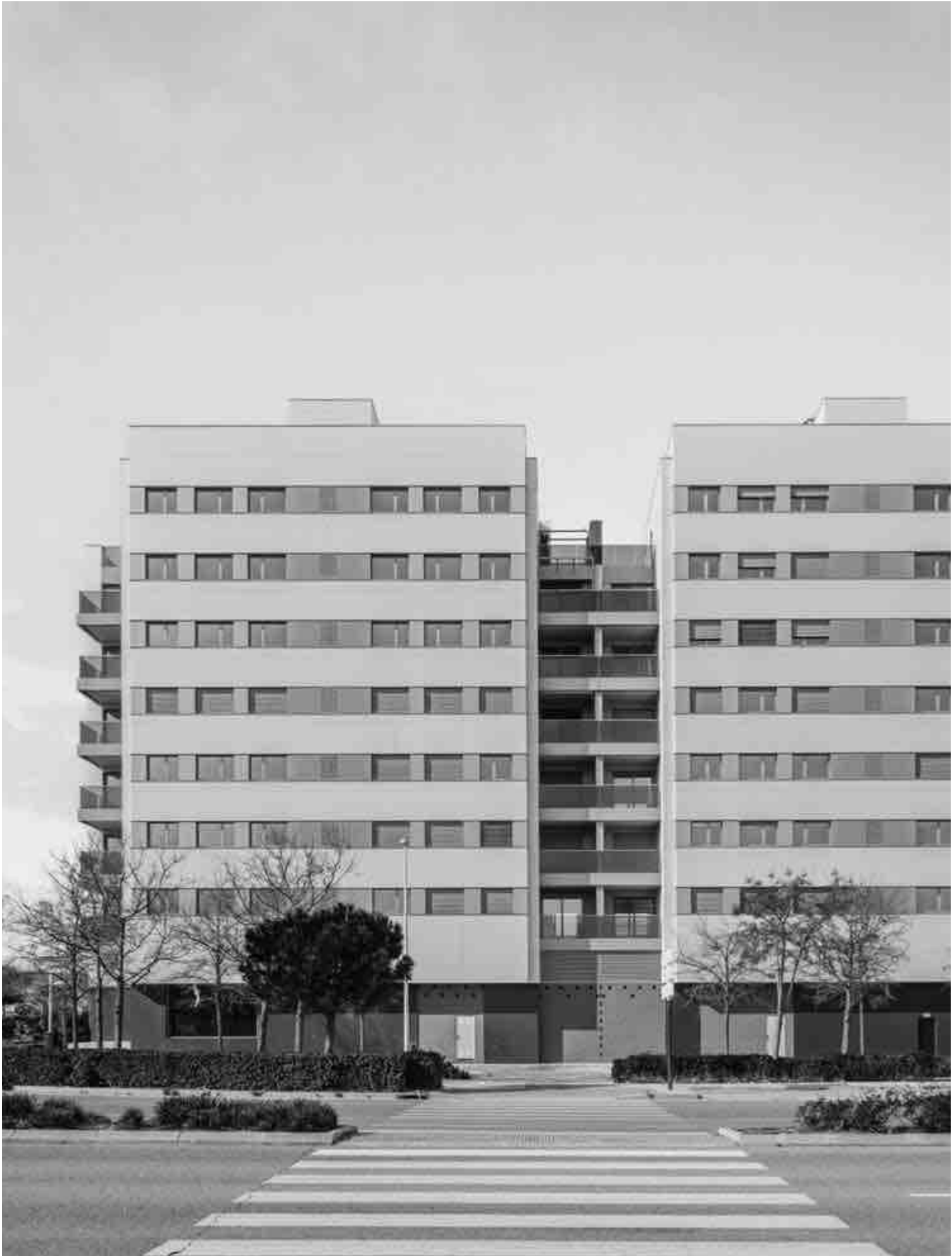
Valdebebas Building, Madrid, Spanje
