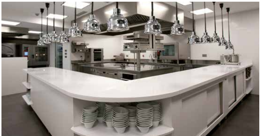
KÜCHE RESTAURANT MUGARITZ / CUCINA RISTORANTE MUGARITZ
