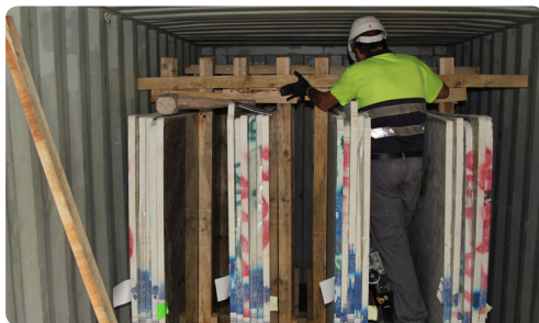
The planks will be nailed to the pallets. Detail of how the safety plank is secured.
