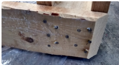
Detail showing how the plank is secured to the base.
