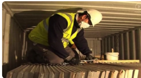
Tensioning the fastening elements to remove knots or twists
