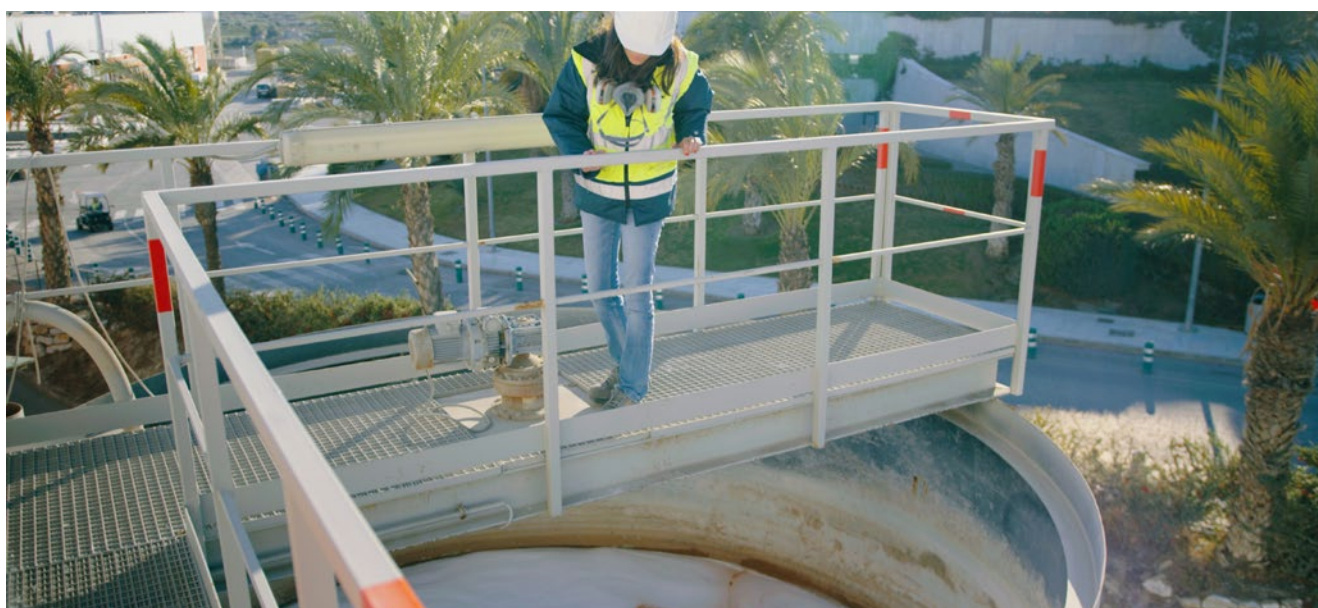
Water Treatment Plant in the Cosentino Industrial Park in Cantoria (Spain)
