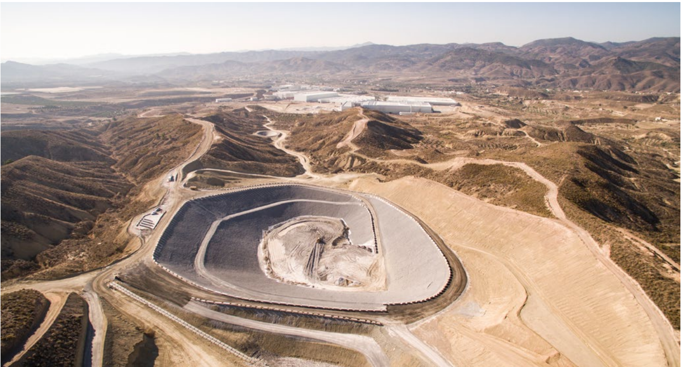
Waste management plant in the Cosentino Industrial Park in Cantoria (Almería, Spain)
