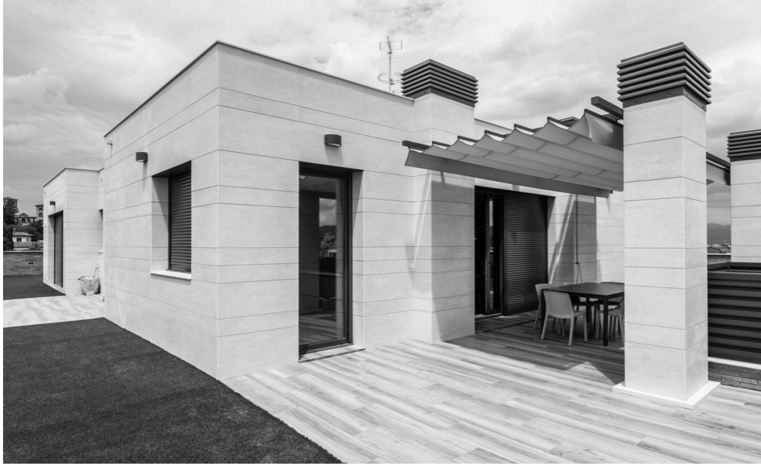
Moles Building, Girona, Spain.
