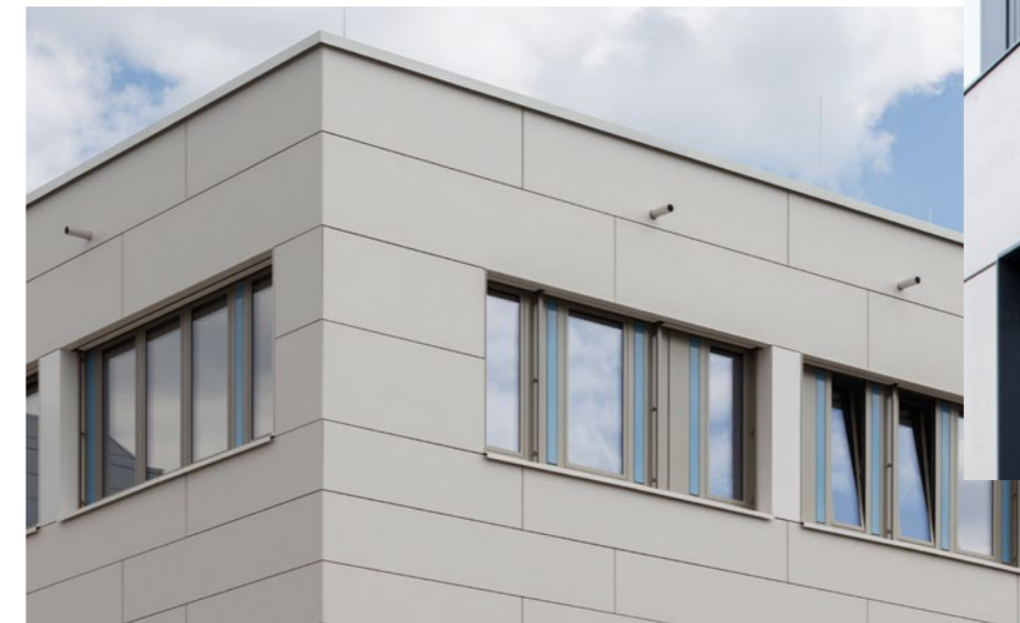
Erlangen Hospital (Germany)
