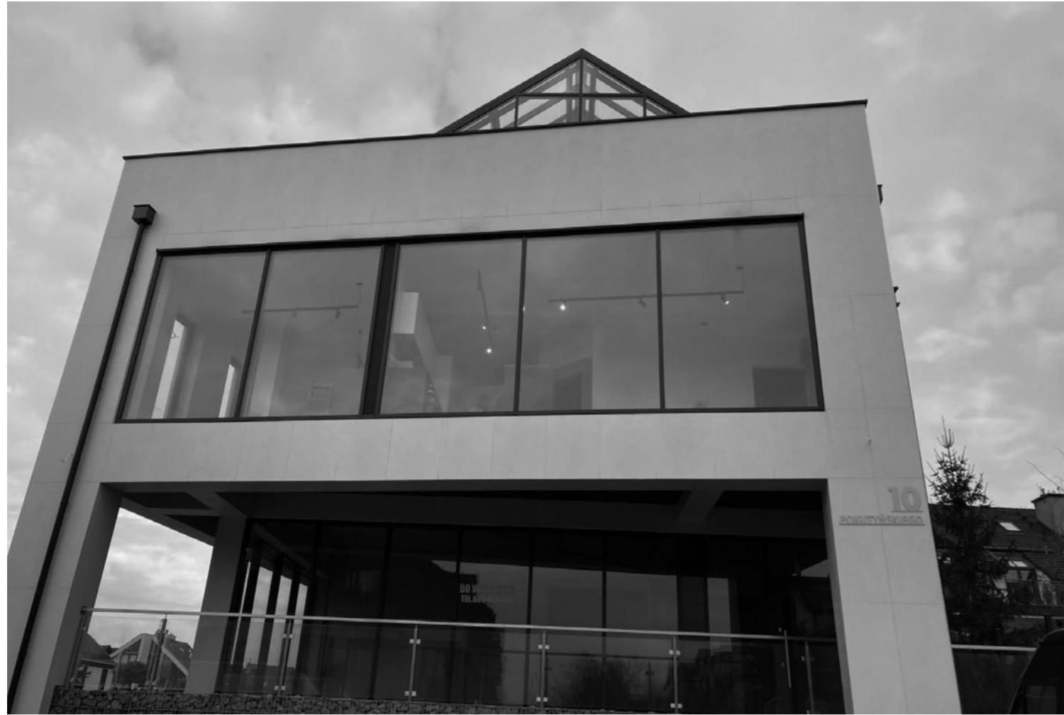
Project with DKS system. Poland
